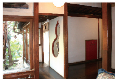
Fire hydrant system in Japanese Inn. Matsumoto-kan
